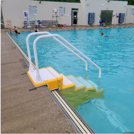
ADA stairs at the outdoor pool
