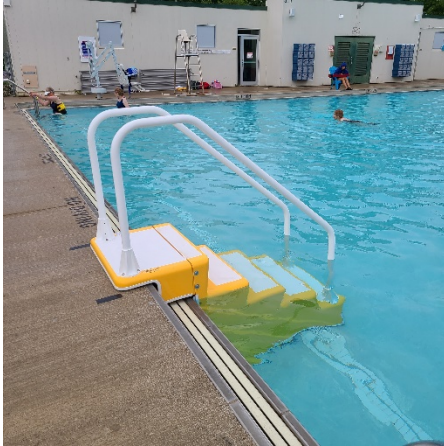
ADA stairs at the outdoor pool
